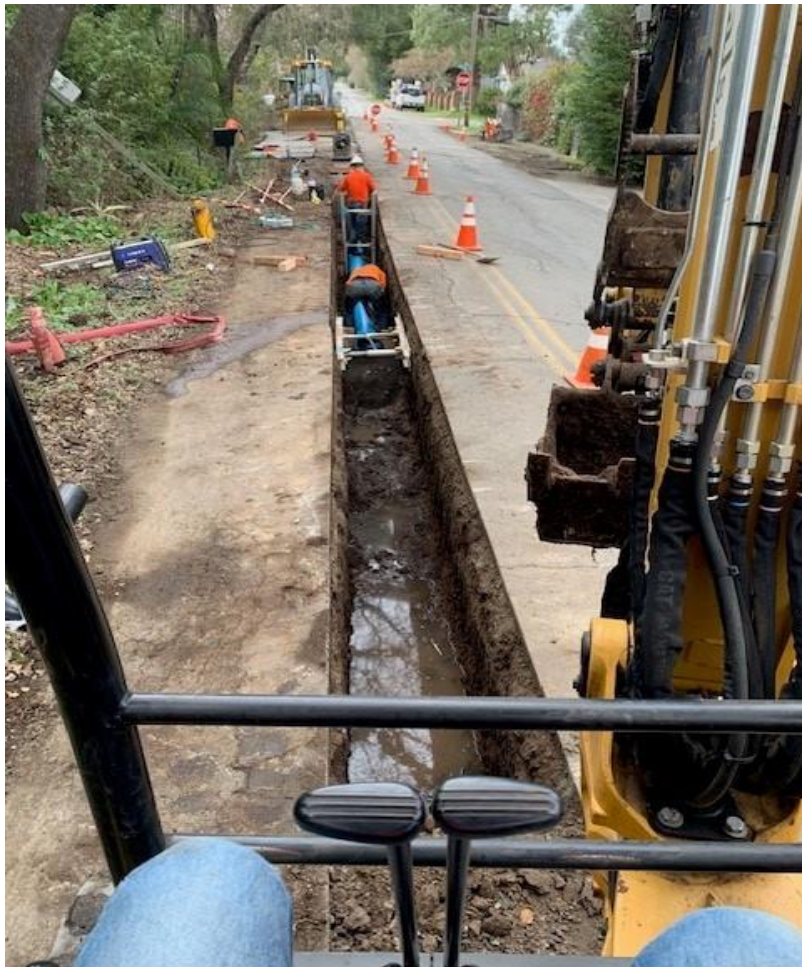
Orange Ave Emergency Main Replacement 02/27/2025
