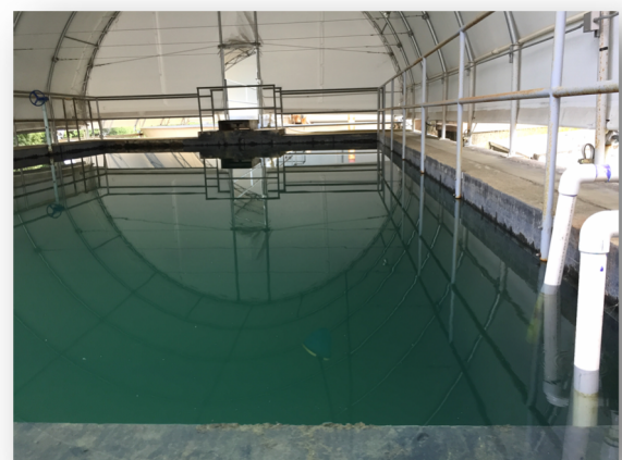
SDC Sedimentation Basin
